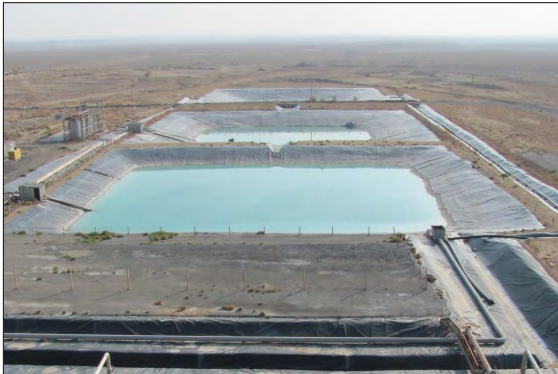
Figure 2-10: Photo of a Pregnant Leach Pond, Intermediate Pond and Barren Solution Pond
